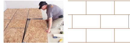
Install Subfloor with Brick Pattern
