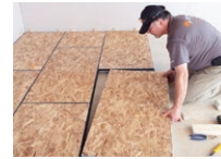
Install Subfloor with Brick Pattern
